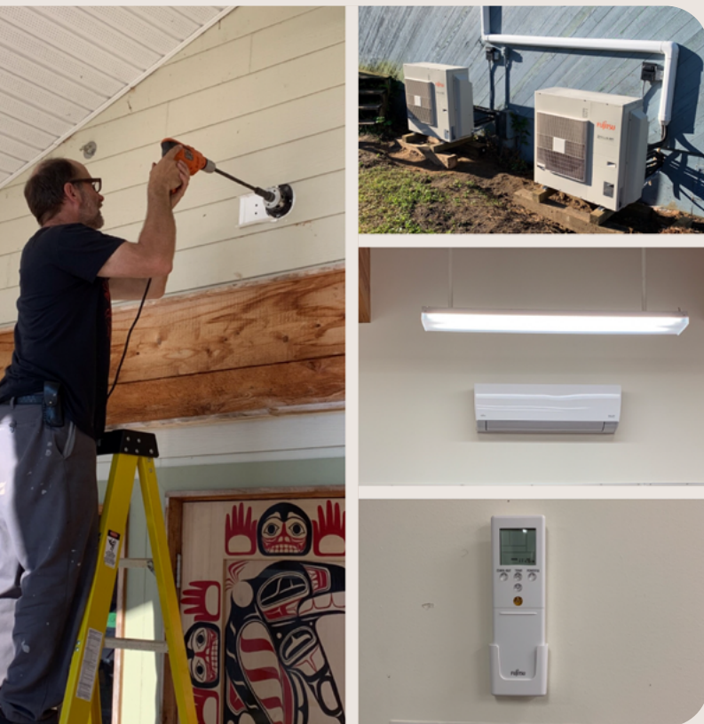
Figure 13 - Heat Pump Installation, Units, and Interior Components
