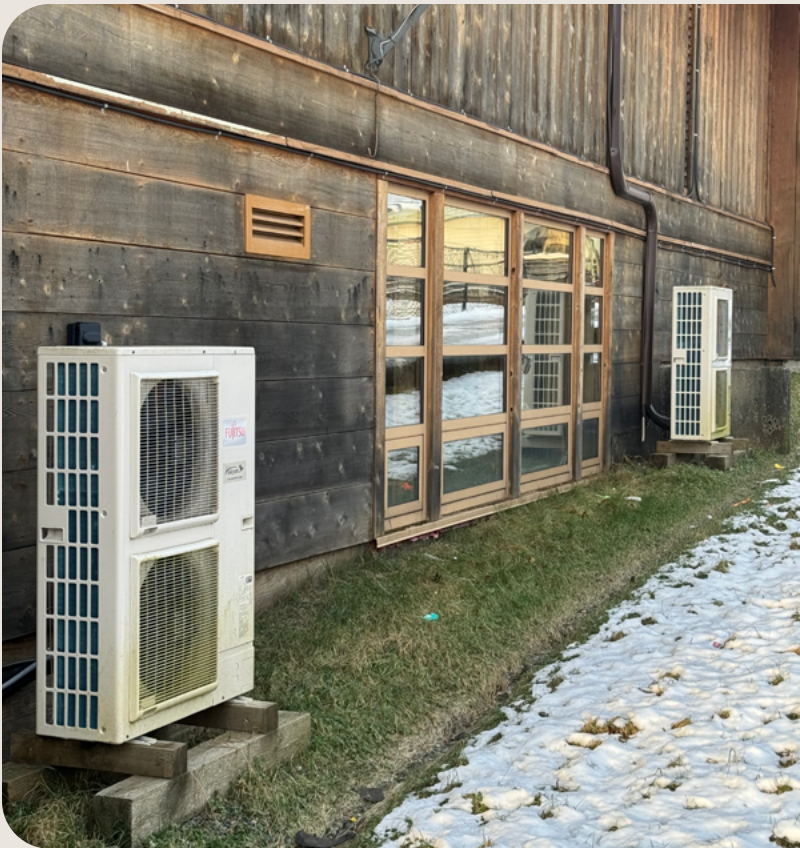
Figure 14 - Heat pumps installed outside of Waaps Wahmodmx
